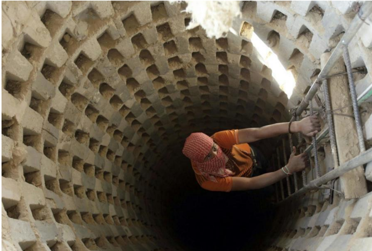
A Hamas operative climbing upward in a pier of one of the major tunnels. Notice the work on the sides of the tunnel.
